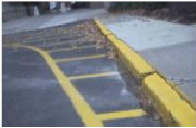
Marked Curb Cut 2.jpg in RGB
